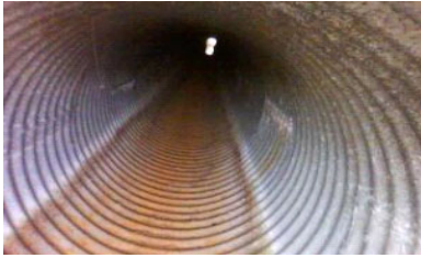
Mild: Minor rust or scaling, no section loss
