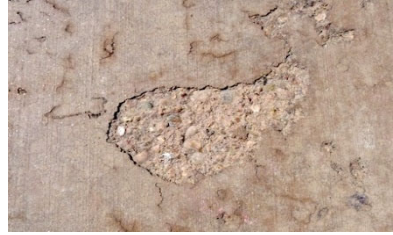
Mild: Minor rust or scaling, no section loss
