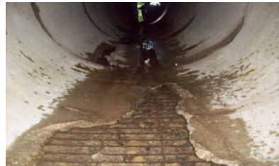
Severe: Complete material section loss (holes)
