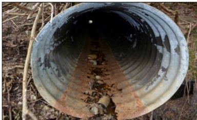
Severe: Complete material section loss (holes)
