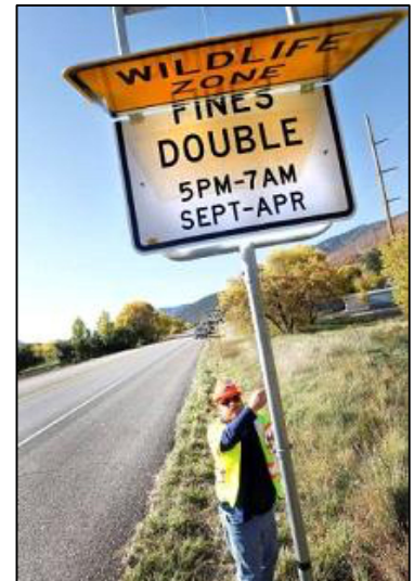
Figure 25. Seasonal wildlife crossing zone sign installed in Colorado that may be folded in half to be concealed. CDOT Photo.
