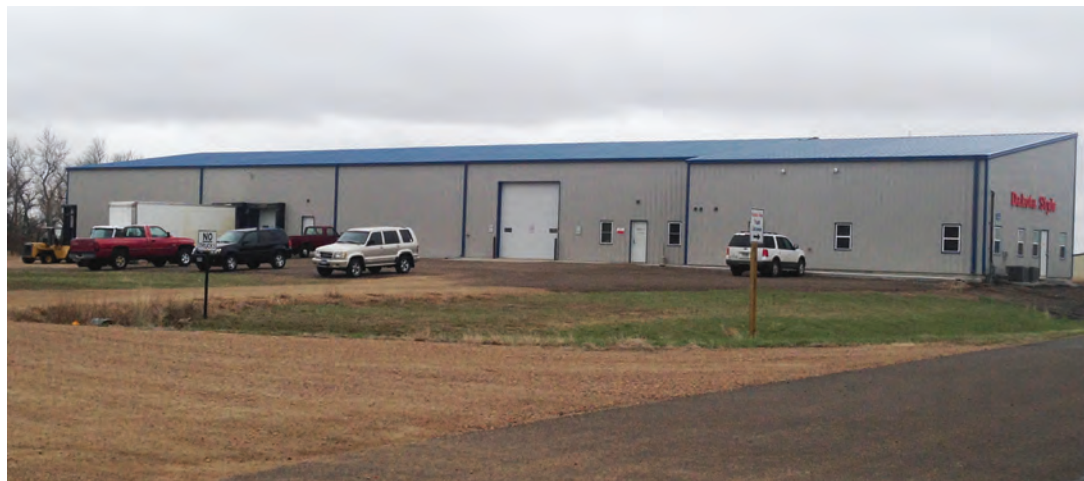
The Dakota Style potato chip and sunflower seed snack plant in the Clark Industrial Park expanded from the dock doors to the left and added office space on the right side.
