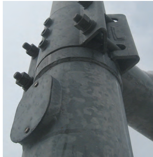
Inspections of lighting and traffic signal poles include the electrical wiring and proper bolting.
