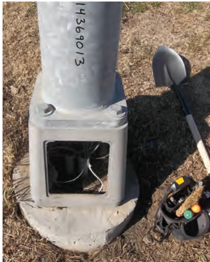
Inspections of lighting and traffic signal poles include the electrical wiring and proper bolting.
