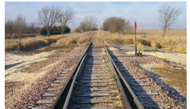
At Napa Junction in Yankton County: the southwest switch on the Platte Line, looking west. Note the overgrown tracks in the distance.
