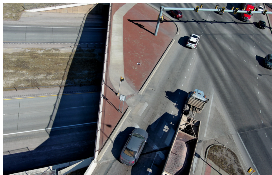
Busy Bridge Intersection
