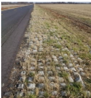
Floodway with reinforced shoulders in Clay County
