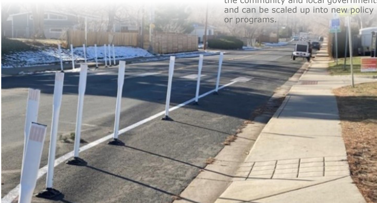
Photo: A Quick-Build Traffic Calming Concept using flexible delineators, slows traffic in advance of a crossing. Source: City of Boulder, CO 29
