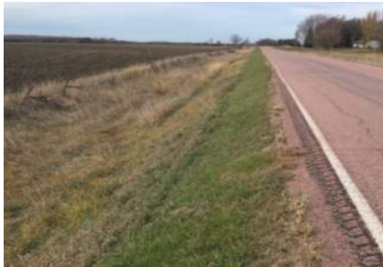
Timber Road: Narrow road, steep inslopes
