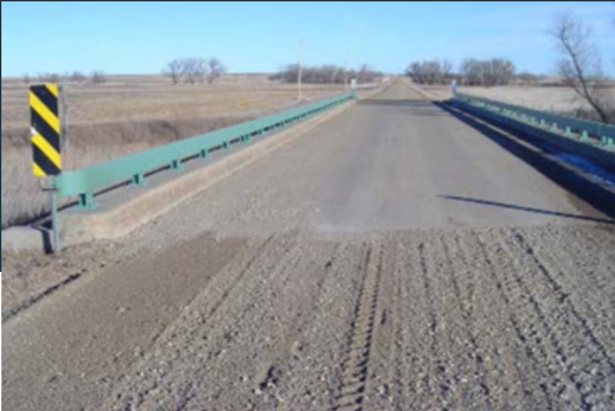
Image of Gravel to Bridge Transition
