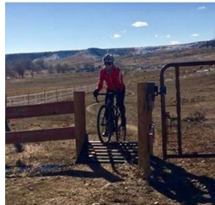
Photo: Example of a ride-over cattle guard on a singletrack trail, this apparatus allows bike and ped access across grazing lands without requiring the use of gates.
