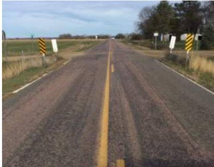
457 Avenue: Narrow road, narrow structure and culvert parapets
