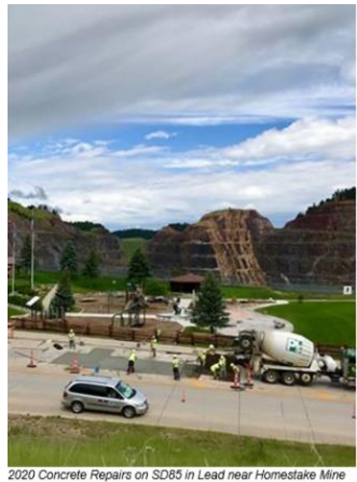
2020 Concrete Repairs on SD85 in Lead near Homestake Mine
