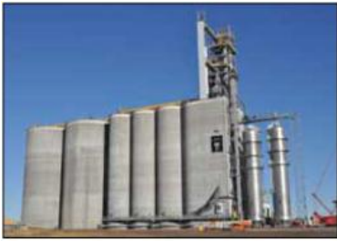
Ground-level view of the new Gavilon elevator nearing completion in early November, one week after a ribbon-cutting open house and already receiving grain. Ground-level photos by Ed Zdrojewski.
