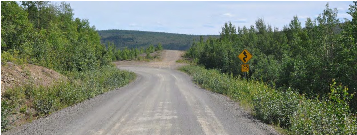
Figure 5. One third of roadway departure fatalities in Tribal areas occurred in a horizontal curve. Photo near the Native Village of Minto shows a visual trap that could lead a driver to miss the curve.
