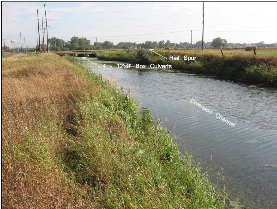
View C-C Looking North along Pelican Lake Diversion Channel
