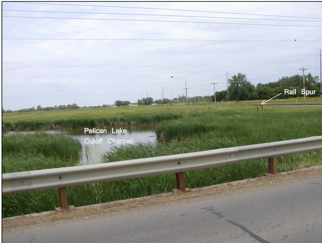
View E-E Looking West from Broadway Street Bridge at Pelican Lake Cutoff Channel
