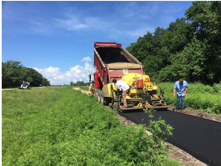
Figure 17: Poor visibility in the morning and evening hours as well as the lack of roadway shoulders made walking and cycling on BIA 500 dangerous. The construction of a separated pathway enhances the safety for motorists and non-motorists traveling this route.
