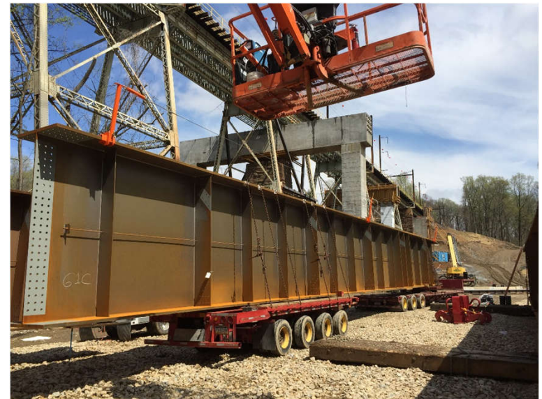
Crum Creek Viaduct, Swarthmore, PA
