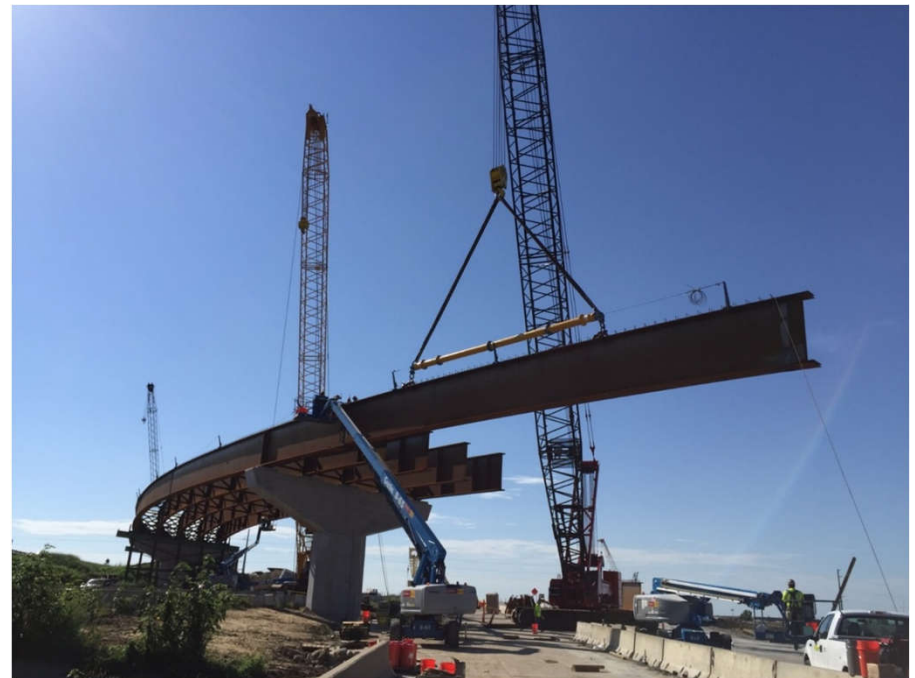
Gateway Interchange Flyovers, Johnson County, KS
