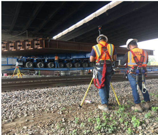
Hole in the Wall RR Bridge, Fort Worth, TX
