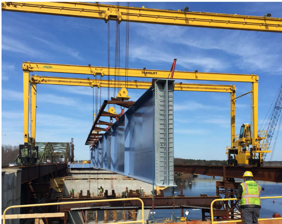
Whittier Memorial Bridge, Newburyport and Amesbury, MA
