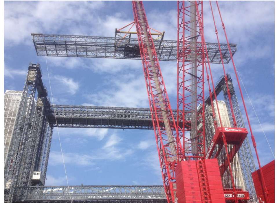
Fore River Lift Span Demolition, Quincy, MA
