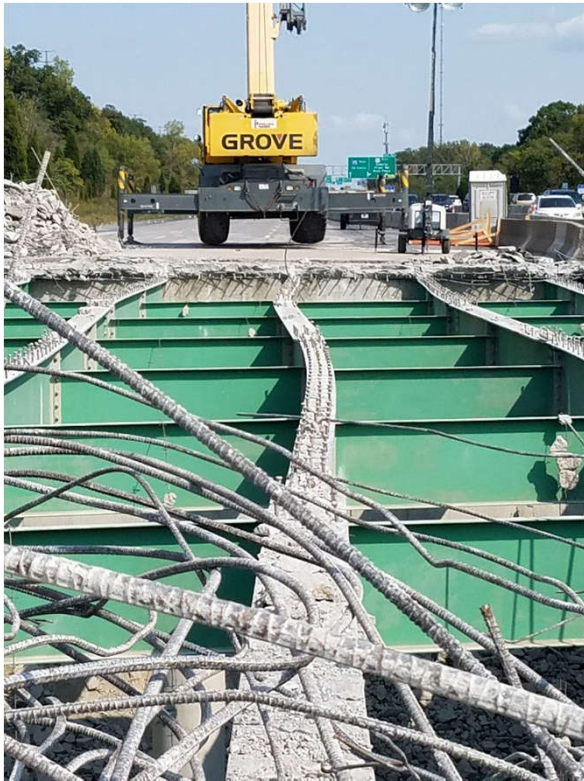
I470 Bridge Re-decking, Kansas City, MO
