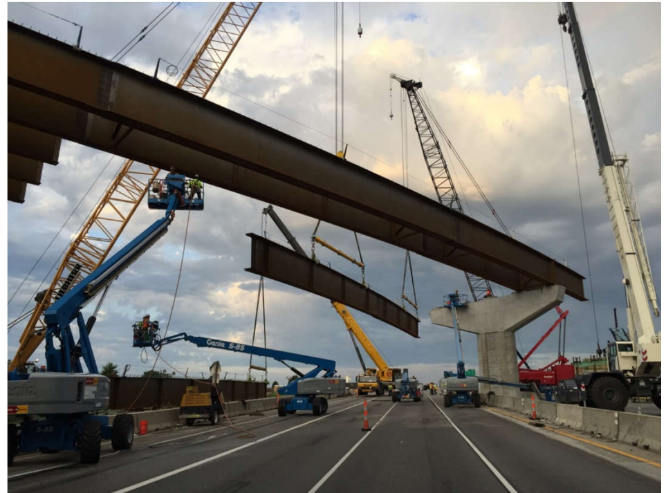
Gateway Interchange Flyovers, Johnson County, KS
