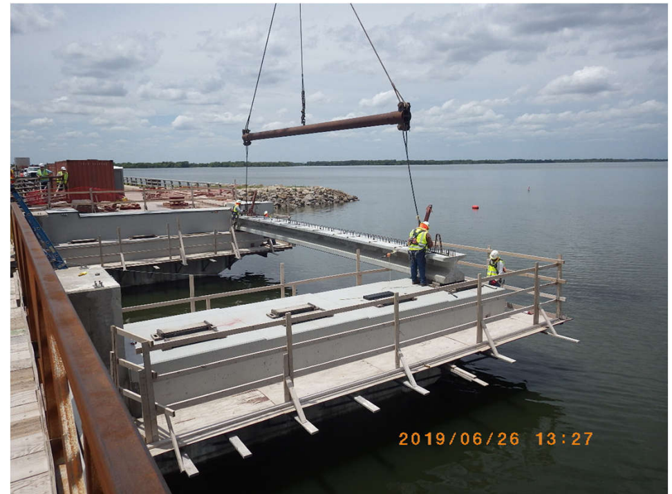
Spillway Bridge, Marion County, KS
