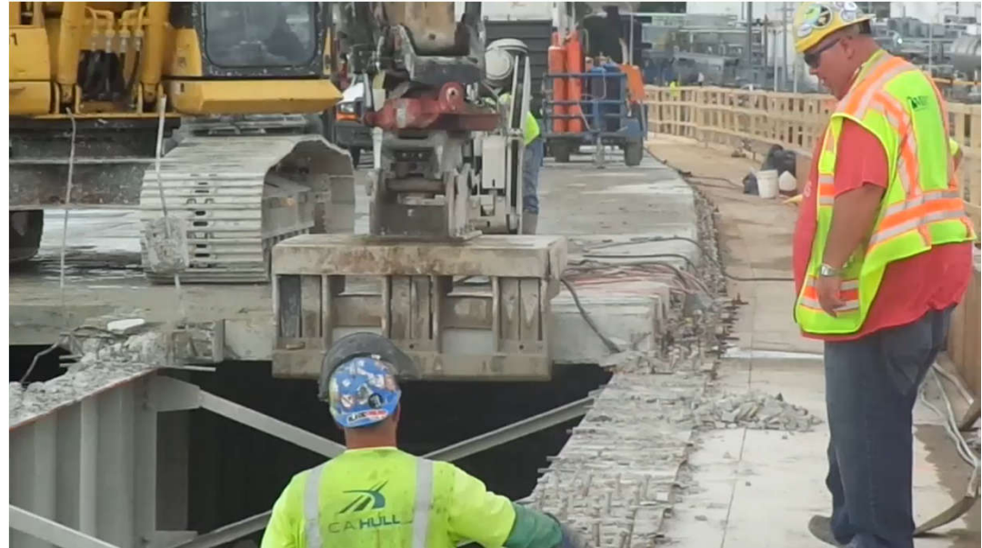
I-75 Deck Replacement, Detroit, MI
