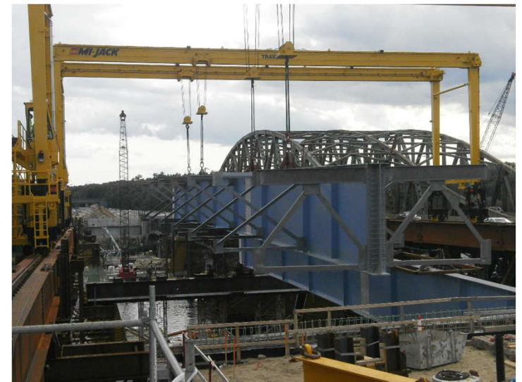
Whittier Memorial Bridge, Newburyport and Amesbury, MA
