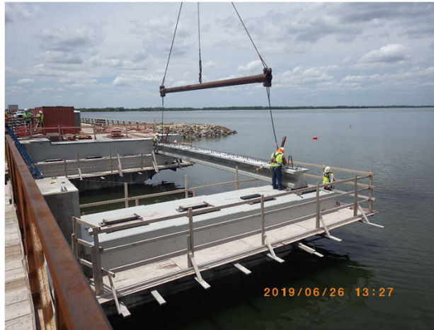
Spillway Bridge, Marion County, KS
