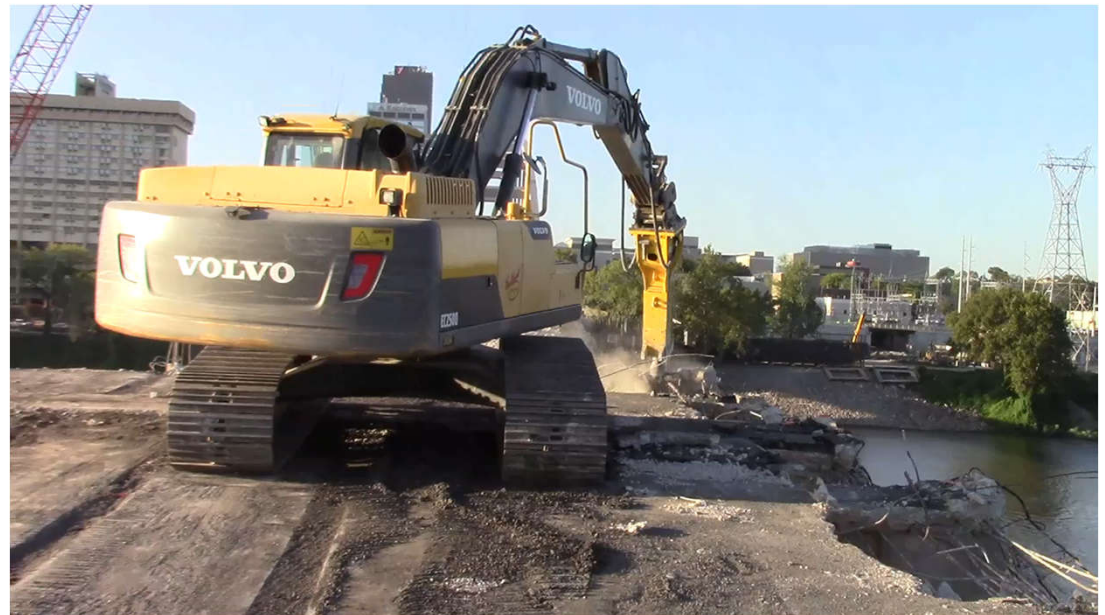
Broadway Arch Bridge Demolition, Little Rock, AR
