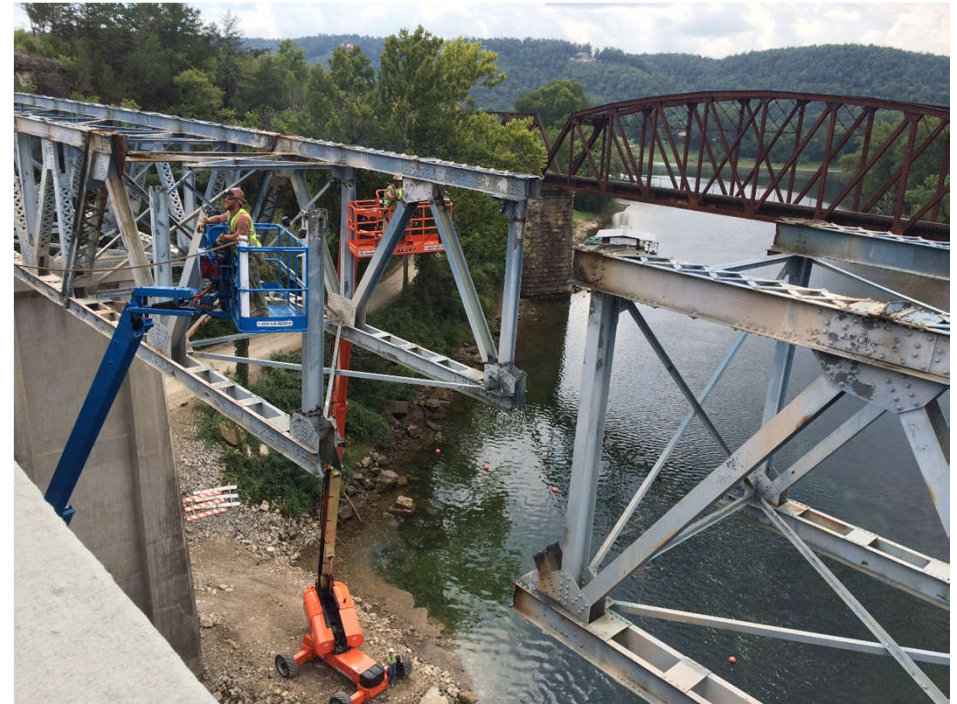
White River Truss Demolition, Prairie County, AR
