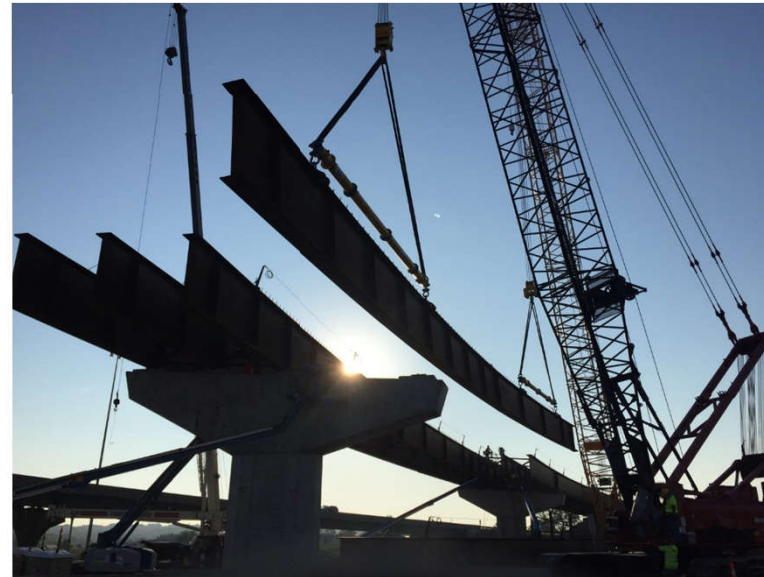
Gateway Interchange Flyovers, Johnson County, KS
