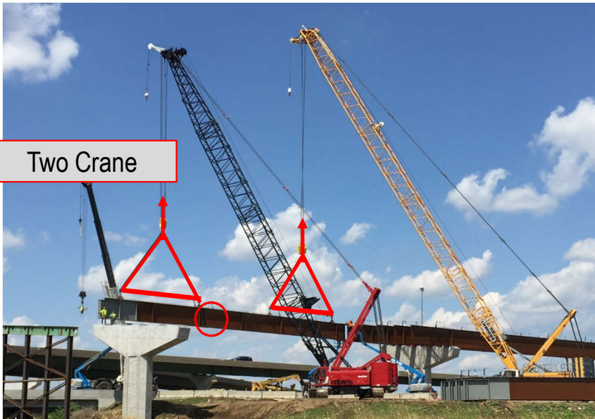
Gateway Interchange Flyovers, Johnson County, KS
