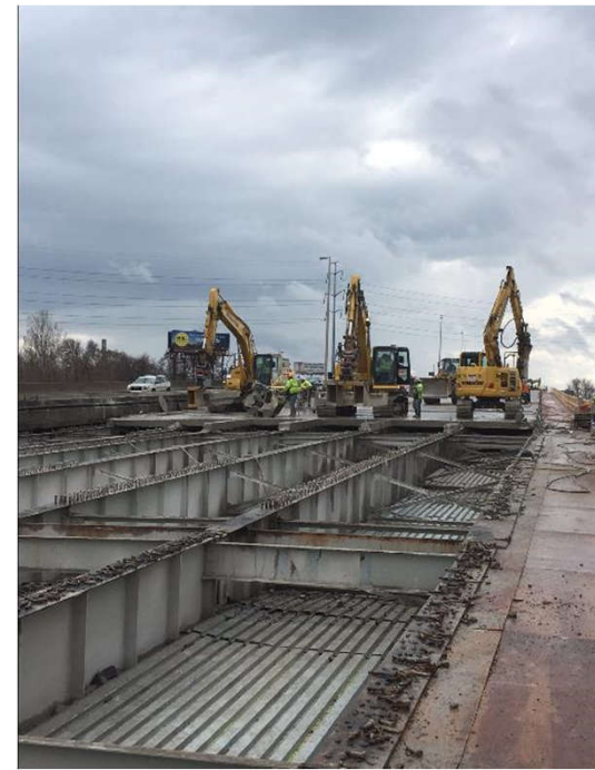
I-75 Deck Replacement, Detroit, MI
