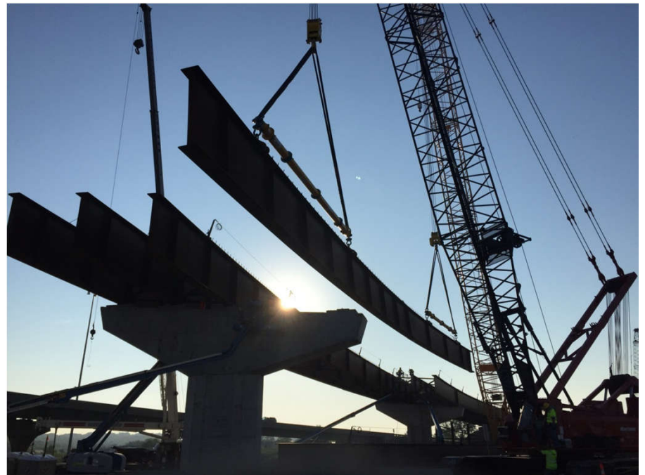
Gateway Interchange Flyovers, Johnson County, KS
