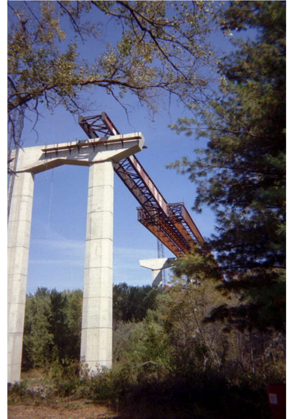
US 20 – Iowa River Bridge
