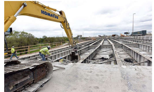
I-75 Deck Replacement, Detroit, MI
