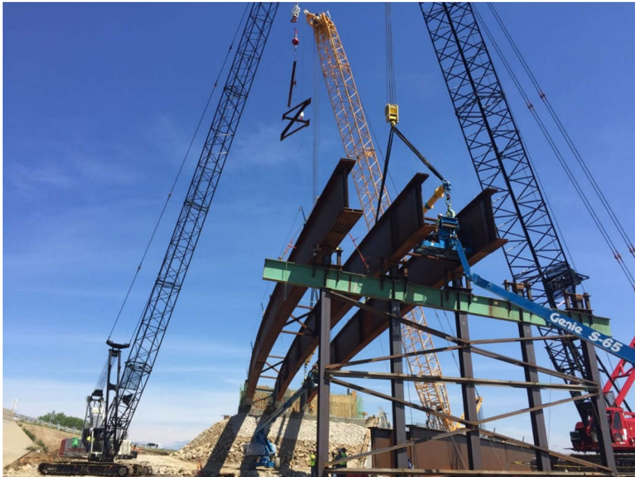
Gateway Interchange Flyovers, Johnson County, KS
