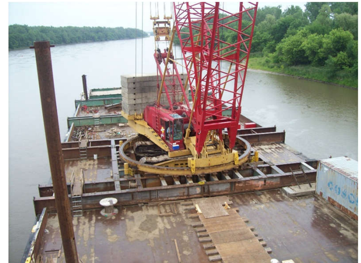
Jensen Construction Ringer, Omaha, NE
