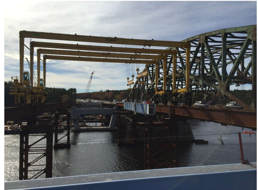
Whittier Memorial Bridge, Newburyport and Amesbury, MA
