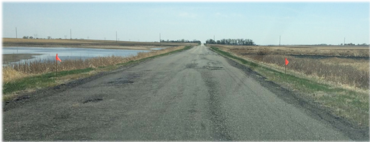
Photo of Pavement Condition of a Brown County Road
