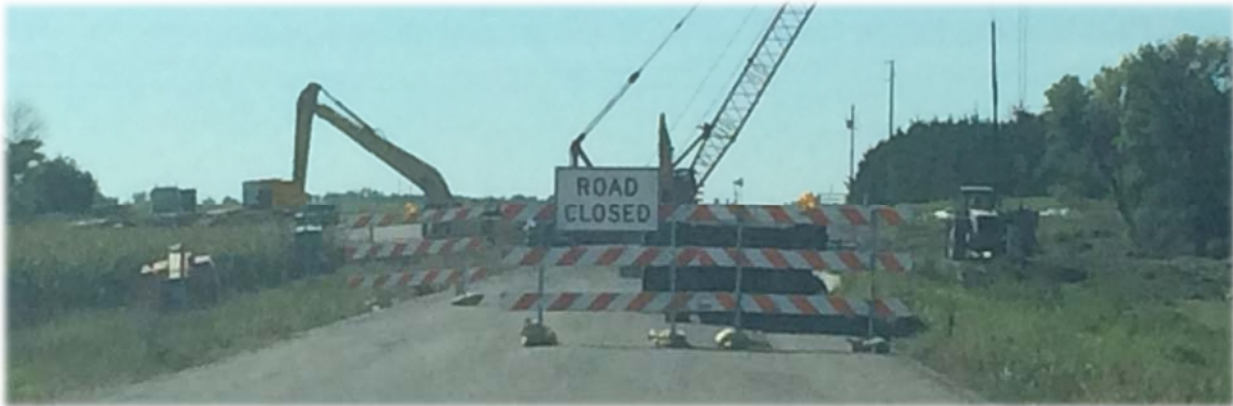
Photo of Construction on a Brown County Road
