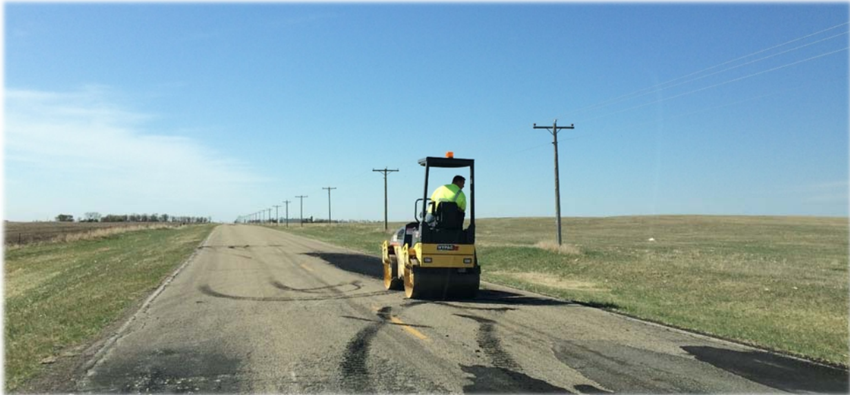
Photo of Maintenance on a Brown County Road
