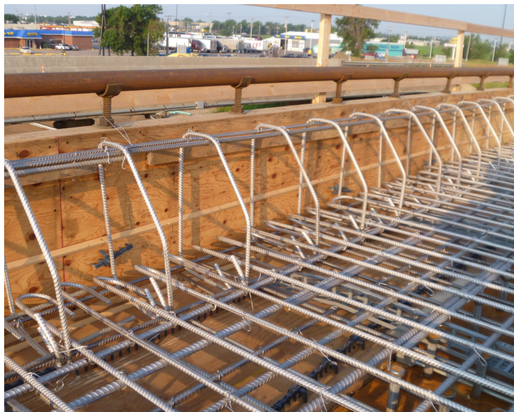
The photo above shows an example of a stainless steel deck.
