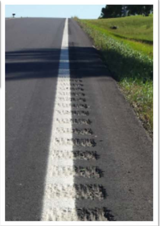
Figure 28: In South Dakota, shoulder rumble strips have shown a 24 percent reduction in fatal crashes, 20 percent reduction in injury crashes, and a 21 percent reduction in roadway department crashes.
