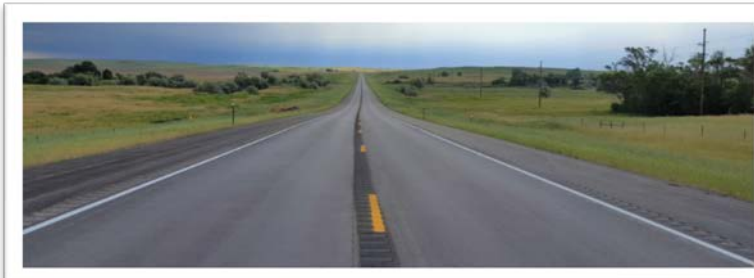
Figure 26: Centerline rumble strips have shown a 50 percent crash reduction.
