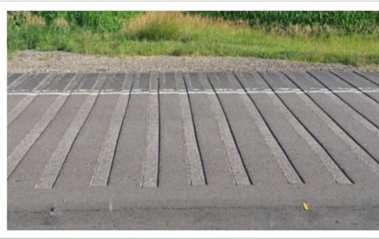
Figure 27: Transverse Rumble Strips provide a 22 percent reduction in injury crashes in South Dakota.
