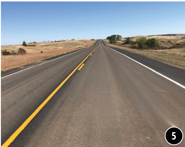
Resurfacing in Central South Dakota A large asphalt resurfacing and pipe repair project between the city of LaPlant to U.S. Highway 83 took place this year. This project included mainline paving, rumble strips, and permanent striping to create a safer driving experience for motorists in the central part of the State.
