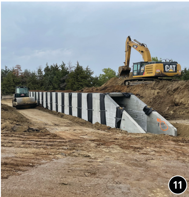
Wide Shoulders Safer Roads A shoulder widening project near Menno on U.S. Highway 18 took the existing 26 foot-wide roadway and expanded it to 36 feet-wide. The goal of this project was to increase the width of the shoulders along the roadway, from one foot to six feet, for safer travel.
