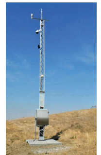
An SDDOT ESS Station.
