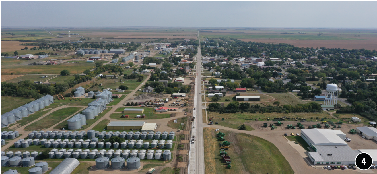
Urban Reconstruction Complete in Gettysburg A two-year, seven phase project to reconstruct U.S. Highway 212 through Gettysburg was completed this year. This urban reconstruction project included grading, storm sewer, new lighting, and better access to local business and parks.
