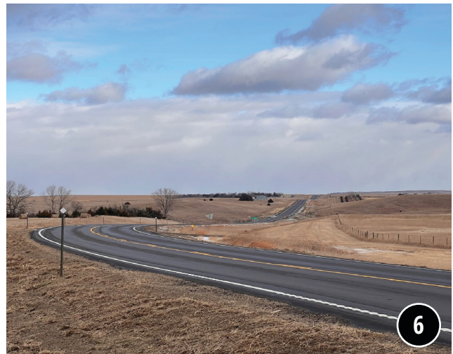
S.D. Highway 49 Receives a Facelift This much-anticipated project on S.D. Highway 49 in Lyman and Tripp Counties created a safer and more enjoyable driving experience for travelers. The project included the repair of several heave areas, pipe repair, and an asphalt overlay.
