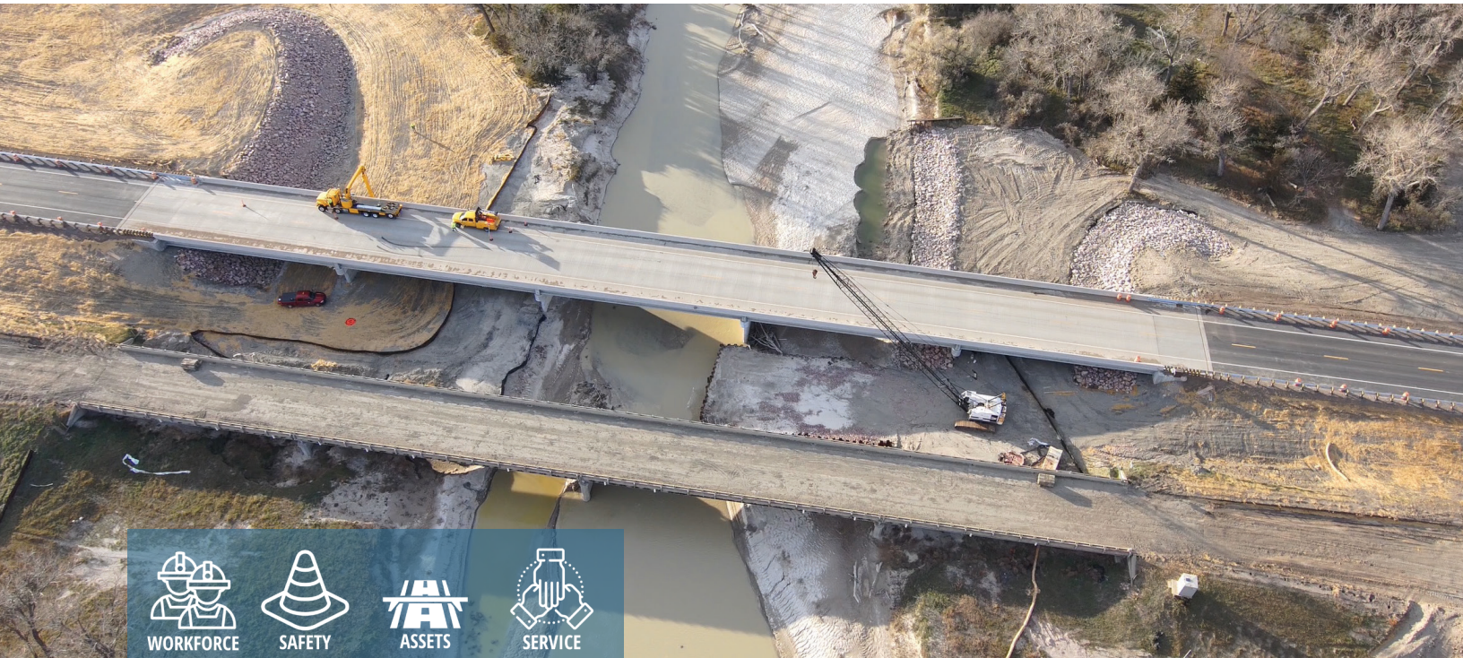
Active construction on U.S. Highway 83.
