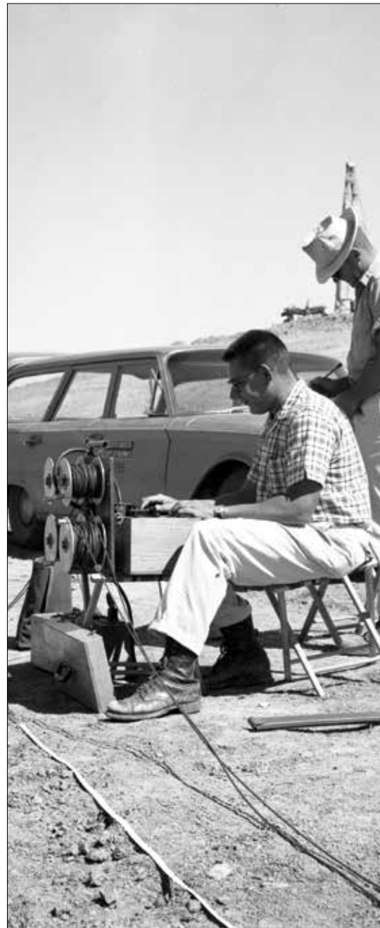
Resistivity testing by department employees in 1963 on a landslide near Interstate Highway 90 in Meade County
