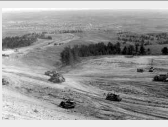
Interstate Highway 90 grading west of Rapid City, circa 1959
