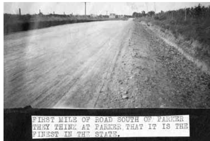
By 1936 standards, a good South Dakota road, graded with a gravel surface
