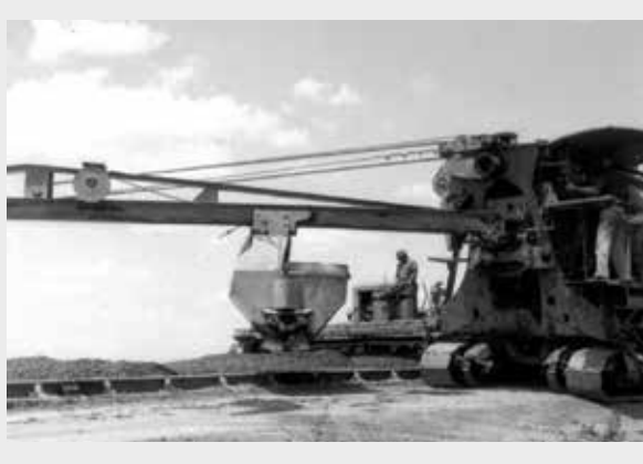
Cement placer on Interstate Highway 29, 1962
