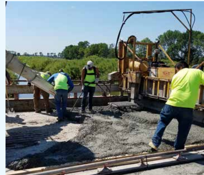
Left: Signs like this one will be posted at completed BIG projects. Right: Construction workers spread fresh concrete over exposed reinforcing steel on the deck of a Brookings County-owned bridge southeast of Bruce. This overlay project was one of four BIG projects completed in 2017.
