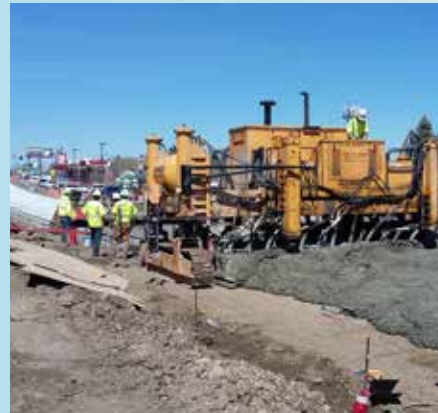
Calined banxite aggregate is spread over pavement previously coated with an epoxy 'glue'. This high-friction surface benefits winter drivers and motorcyclists navigating the Black Hills' many winding roads.
