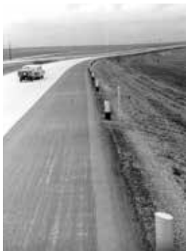
Above: Posts along Interstate Highway 90 in Pennington County, 1964. Right: Cable guardrail on I-90 in 2017.
