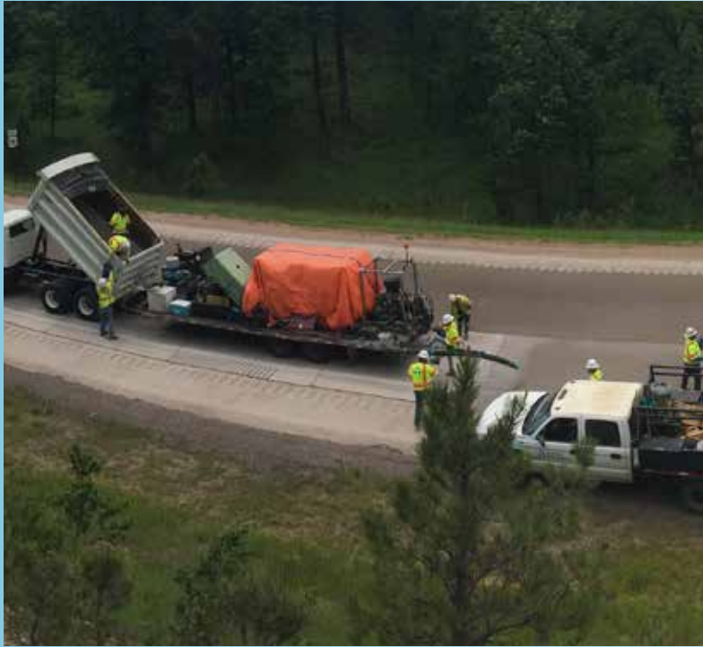
Calined banxite aggregate is spread over pavement previously coated with an epoxy 'glue'. This high-friction surface benefits winter drivers and motorcyclists navigating the Black Hills' many winding roads.
