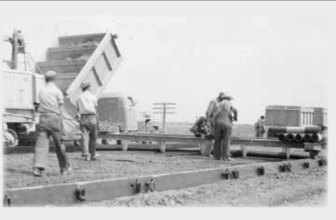
1947 photograph of "manner of laying subgrade paper with special cart"
