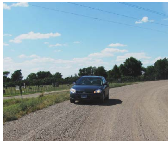
Well-shaped superelevation on a curve.
