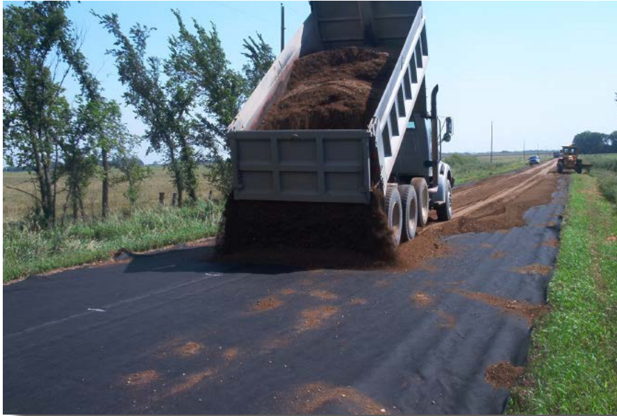
The same road being repaired during summer construction season by shaping the existing road and placing a geotextile fabric on the surface. Placing a minimum thickness of 6-inches in the first layer over fabric is generally recommended.
