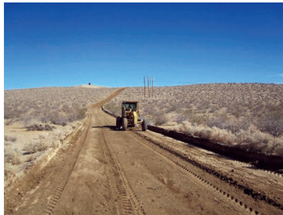
Grading is the primary maintenance performed on unpaved roads (Source: Envirotac).
