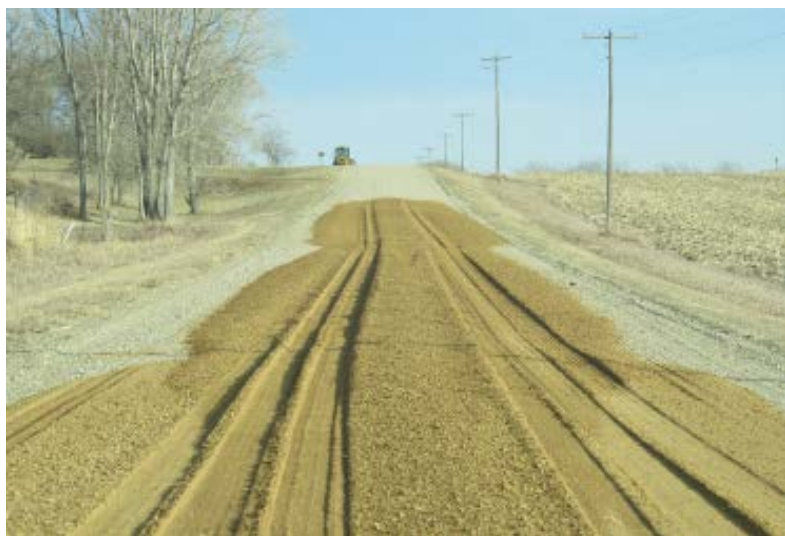
A good example of evenly dumping gravel on the road. Notice a grader is ready at the hilltop to begin processing the gravel.
