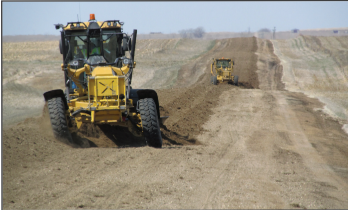
Reconstruction work space. (Source: Greg Vavra, SDLTAP).
