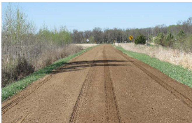
A well-prepared road surface ready for treatment.
