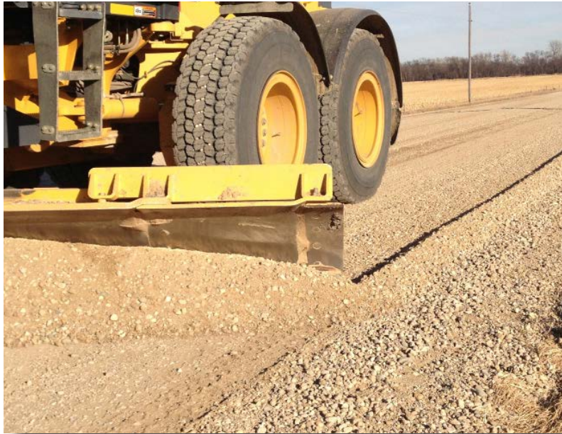
If leaving a maintenance windrow is allowed by policy, this is a good example of a light windrow being placed at the edge of the roadway.
