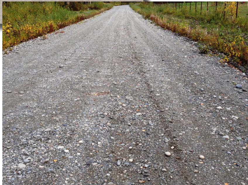
These roads show a remarkable contrast in surface condition due to quality of surface gravel.
