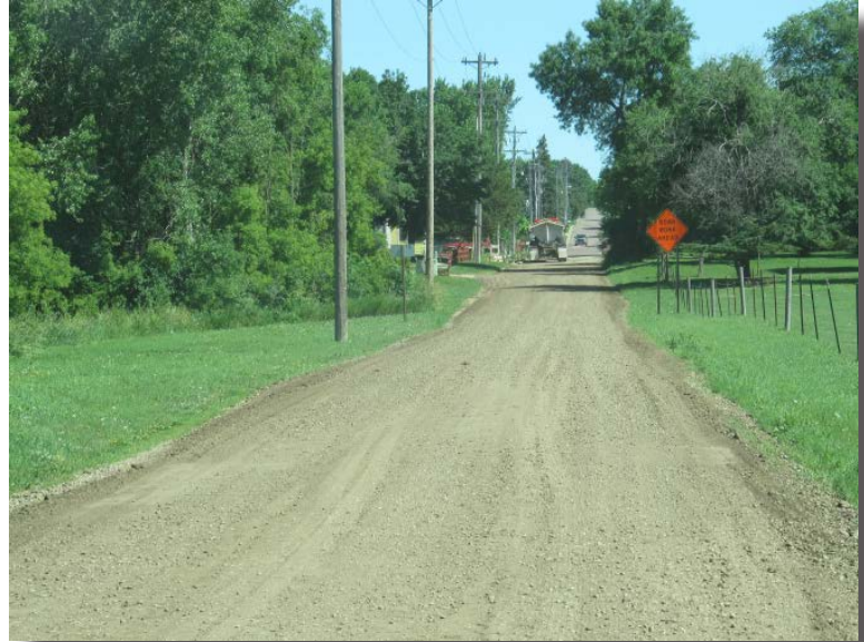
Example of mixed recycled asphalt and surface gravel used on a road with very low traffic.
