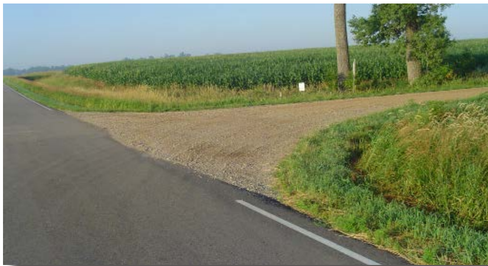
A well-shaped intersection of gravel surface and paved road.
