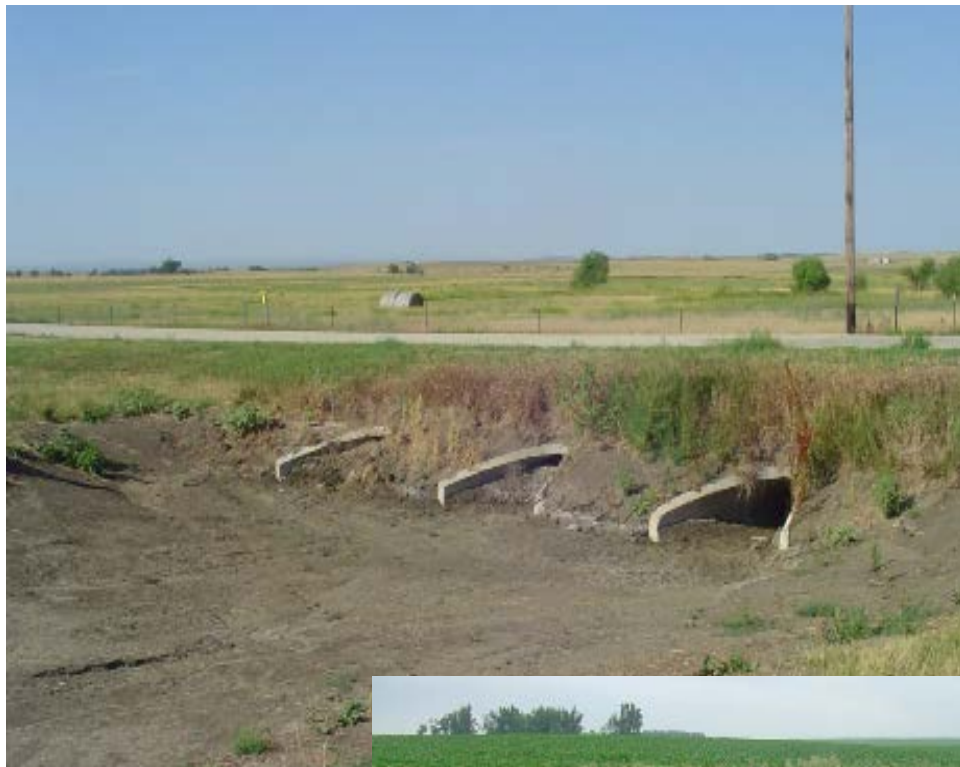
Good work in progress to clean soil from ditch and existing culverts.
