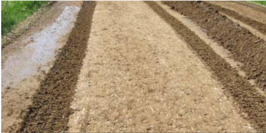
It is a good practice to loosen, mix and reshape gravel in a washboard-prone area while it is moist.
