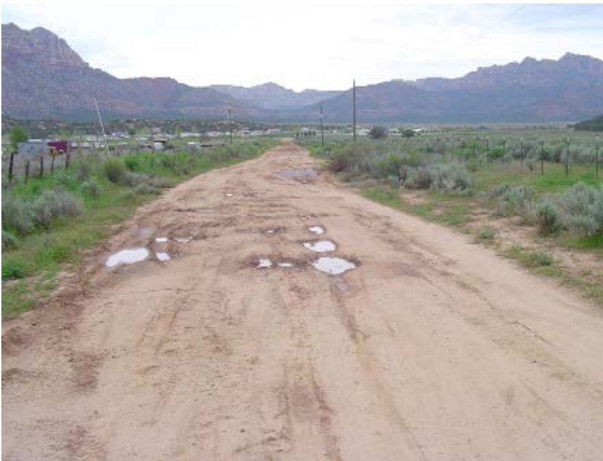
This road, located in a desert region, performs poorly even though the average annual precipitation is less than 10 inches per year.
