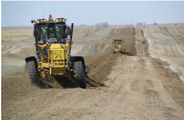
Reconstruction work space. (Source: Greg Vavra, SDLTAP).
