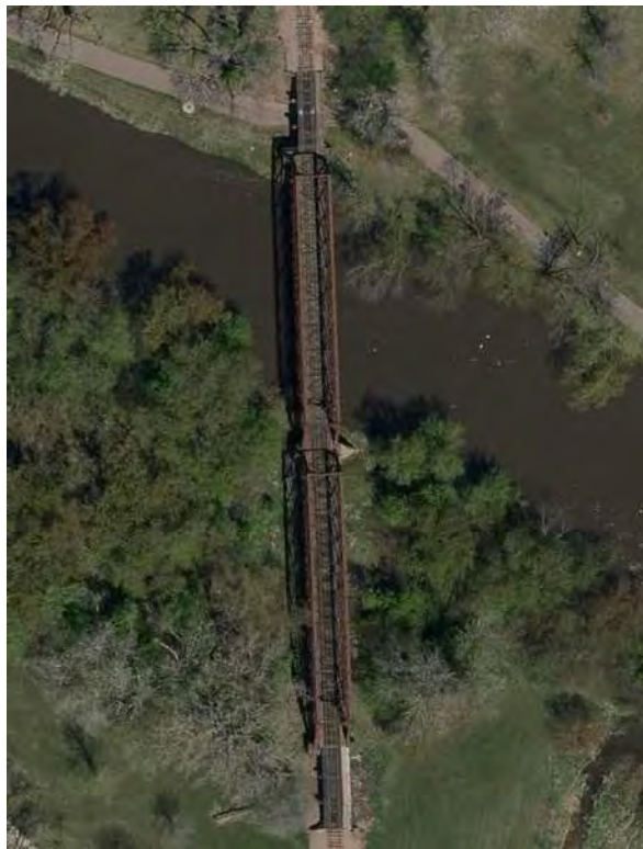
Figure 14. Satellite view of Bridge P125.
