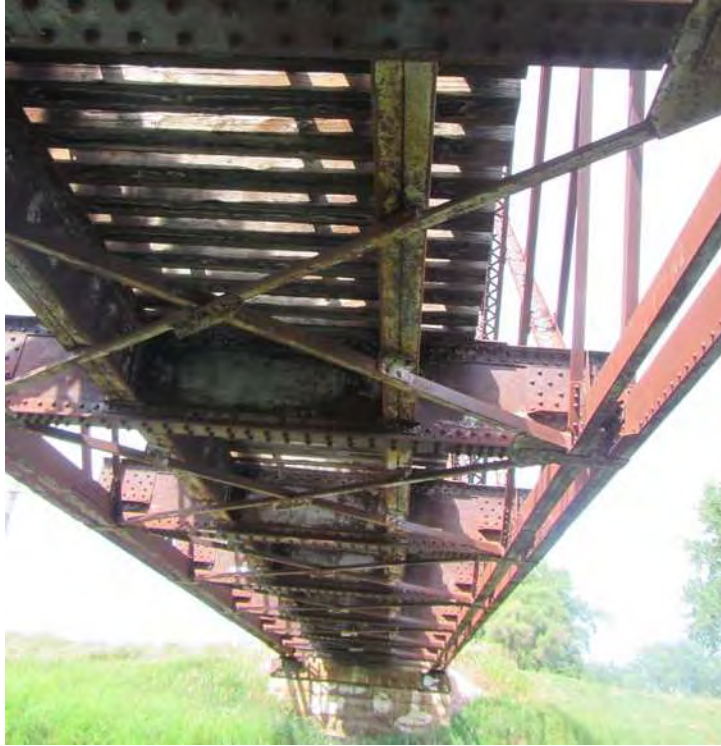
Figure 25. View of steel truss deck, Bridge P131, facing west.
