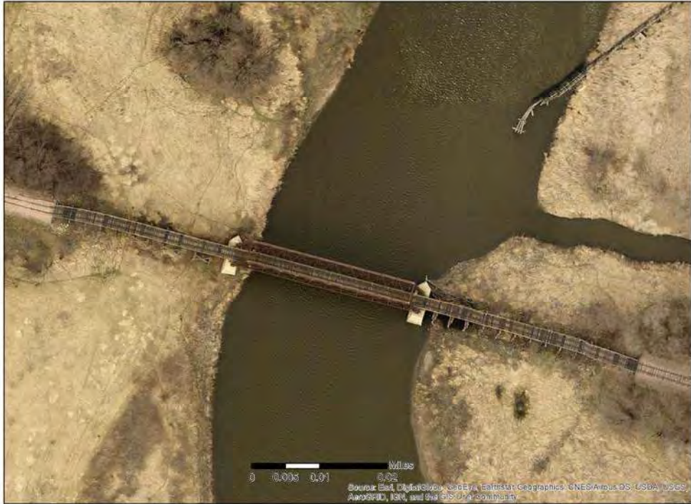
Figure 7. Satellite view of Bridge P106.
