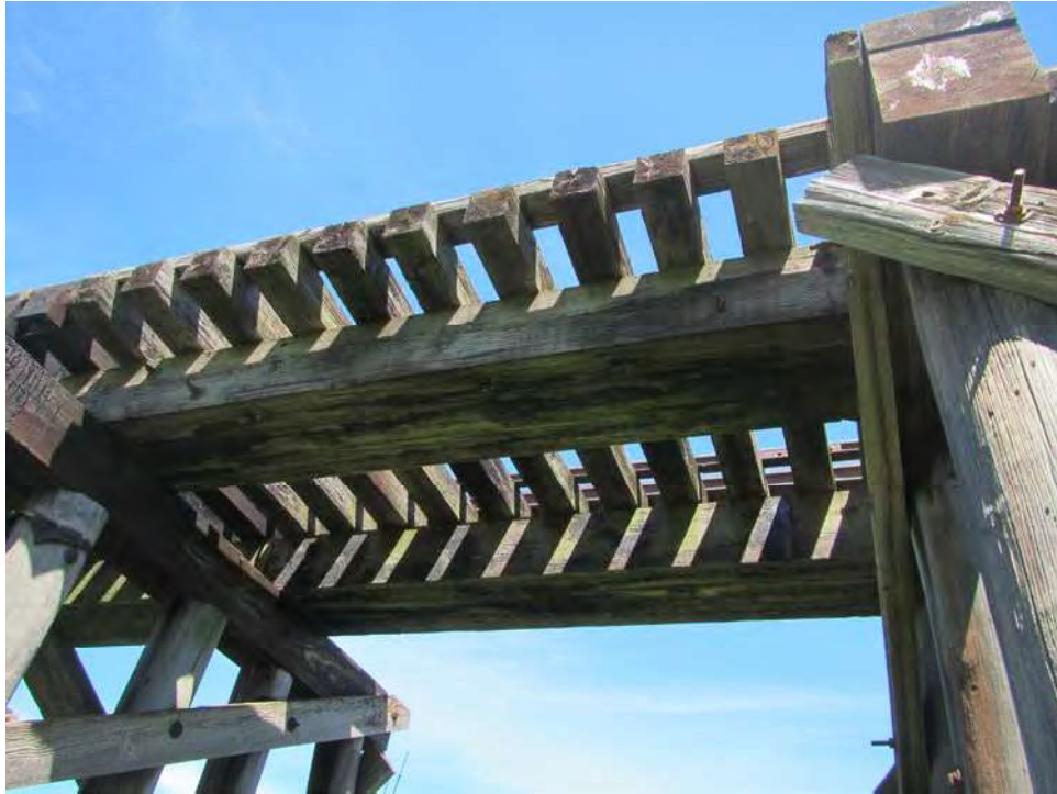
Figure 11. View of Bridge P106 trestle deck from beneath, facing north.
