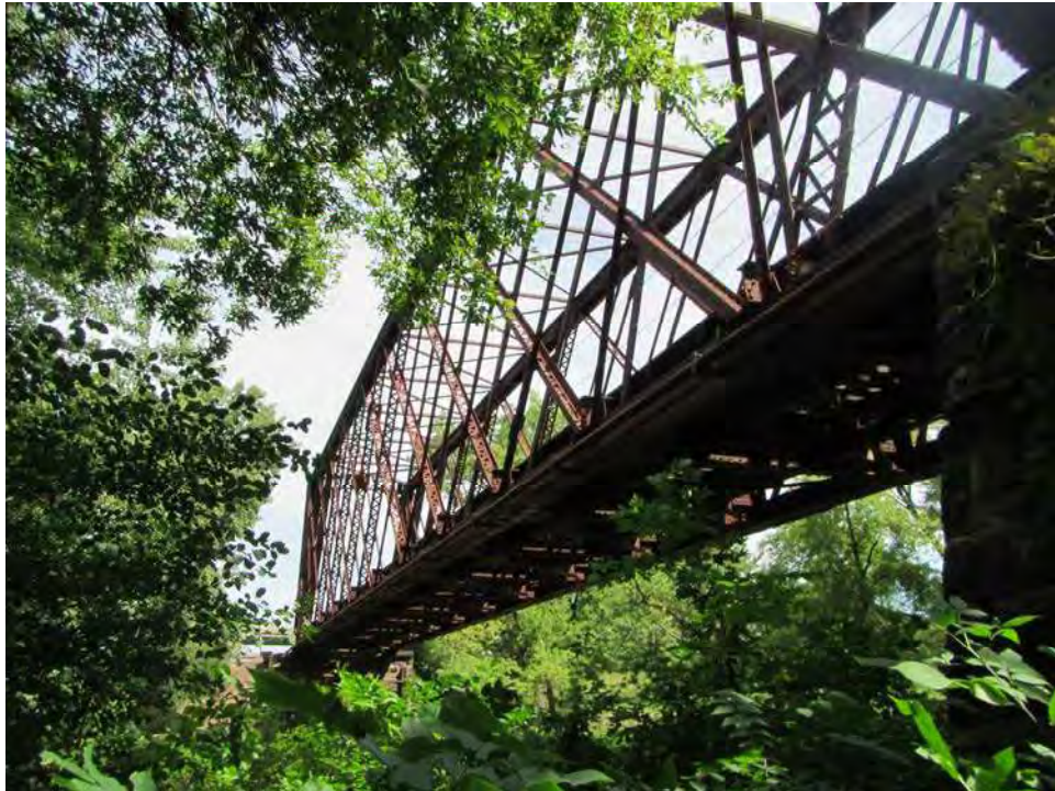
Figure 18. View of northern half of Bridge P125 truss structure, facing north-northeast.
