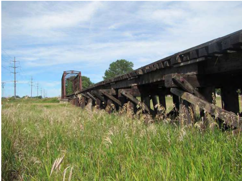
Figure 22. View of timber trestle approach structure, Bridge P131, facing west-northwest.
