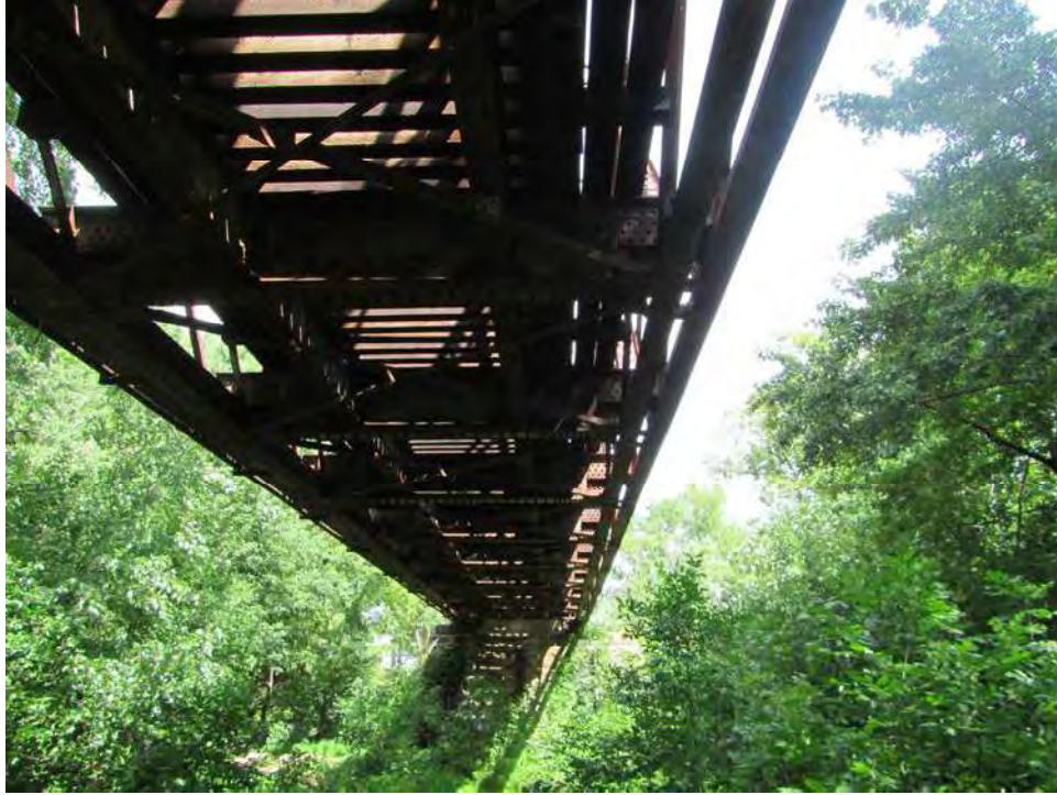
Figure 17. View of Bridge P125 truss deck from beneath, facing north.
