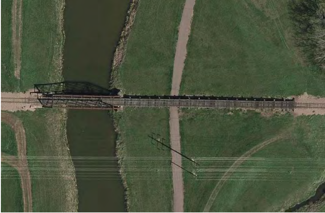
Figure 19. Satellite view of Bridge P131.
