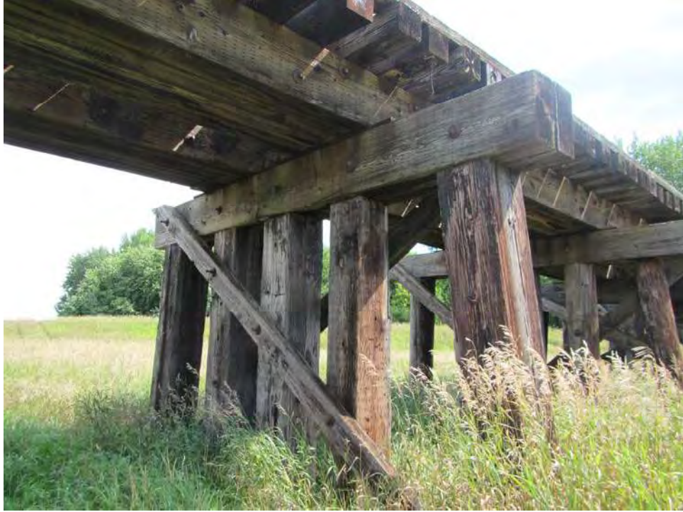
Figure 23. View of timber trestle support structure, Bridge P131, facing northeast.
