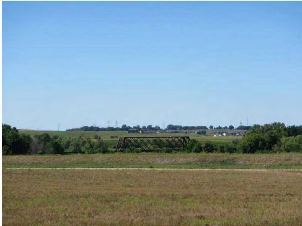
Figure 8. Overview of the Bridge P106 project area, facing southwest.
