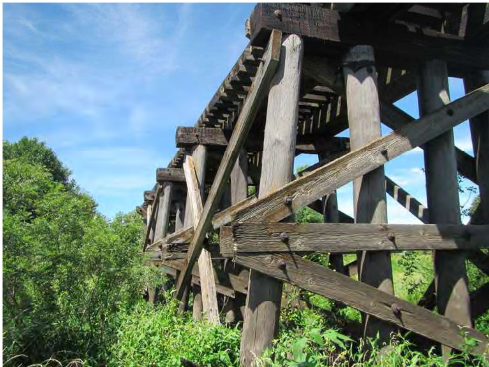
Figure 12. View of timber trestle approach, Bridge P106, facing west.
