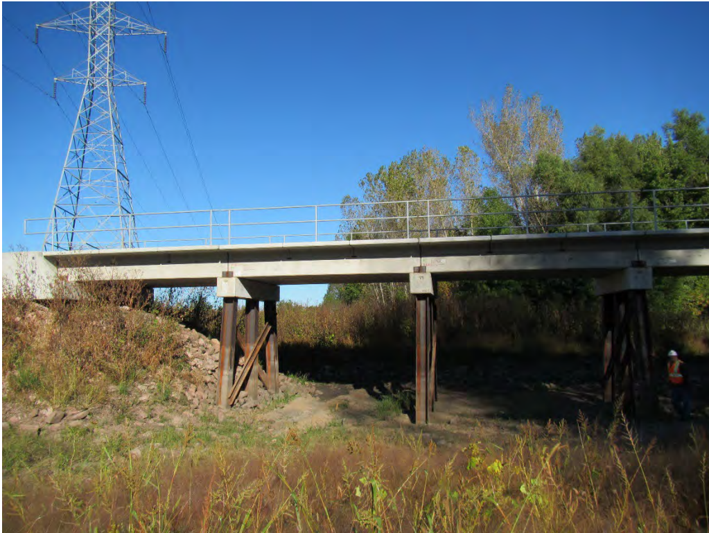
Profile view of the replacement materials at Bridge T-478.
