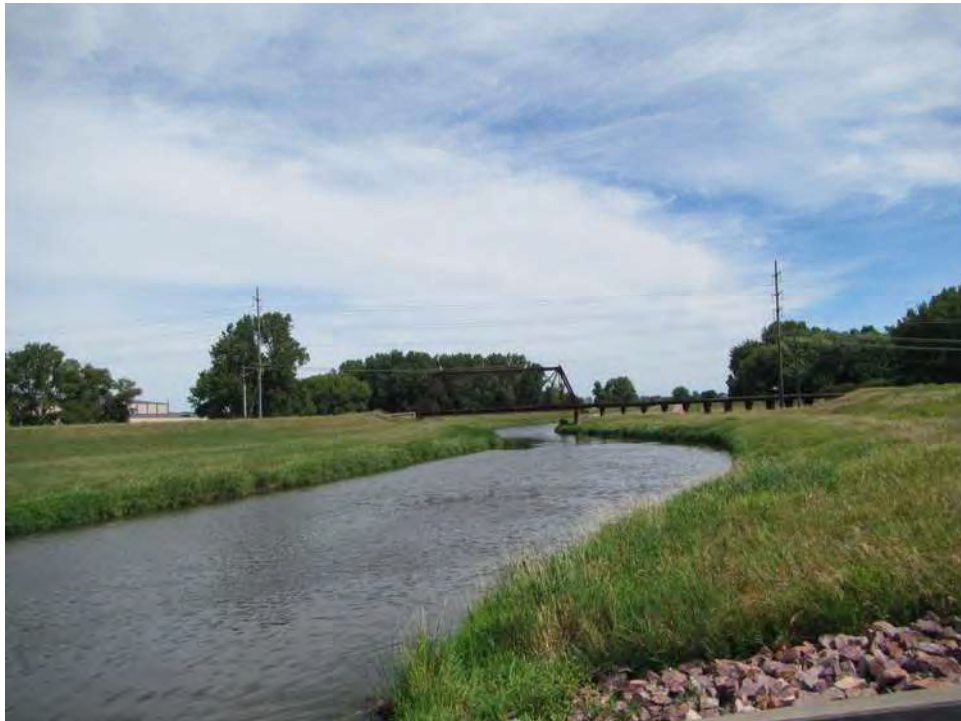
Figure 20. Overview of Bridge P131, facing north.
