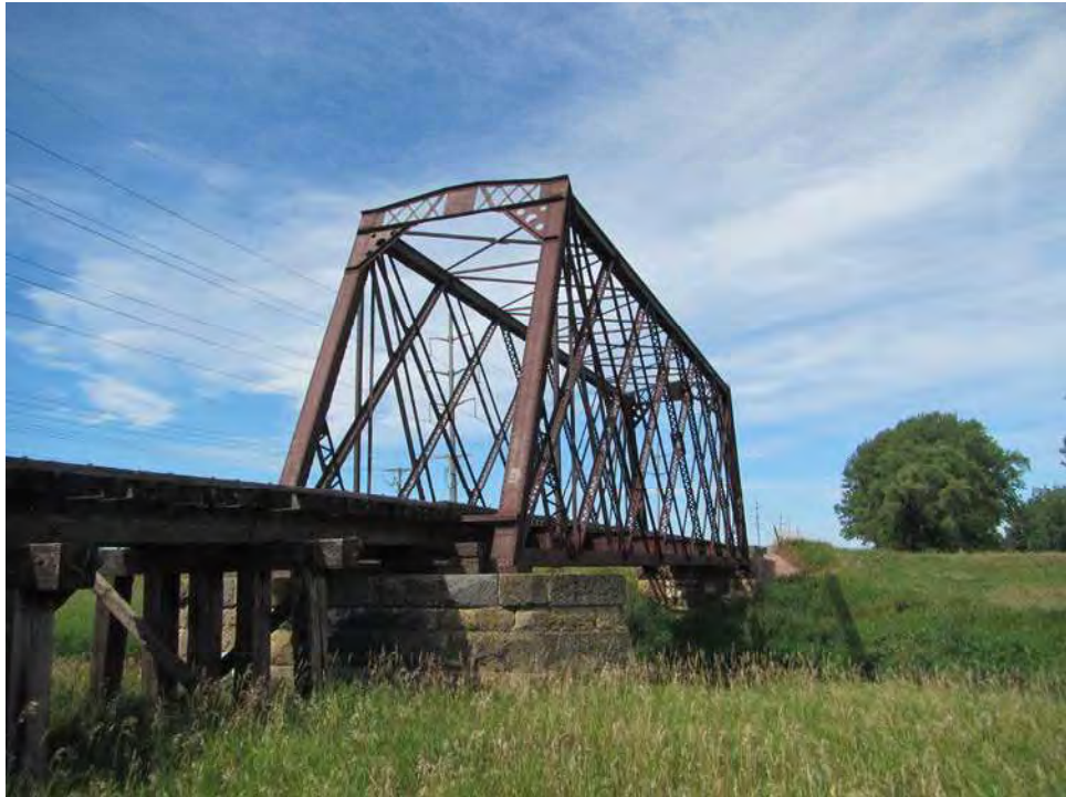
Figure 24. View of steel lattice through truss, Bridge P131, facing southwest.
