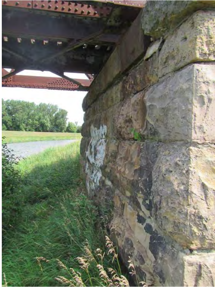
Figure 27. Close-up opposing view of support column in Figure 26, facing north.
