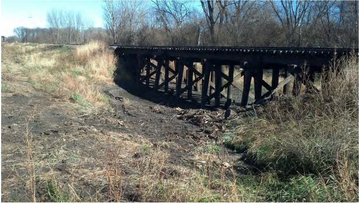
View of timber trestle Bridge T-478.
